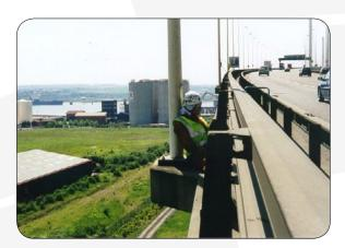
QEII Bridge (cable-stayed bridge opened in 1991) ACFM<sup>®</sup> inspection of lamp post welds.
